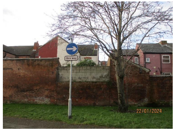
Rear of site viewed from Regent Street.
