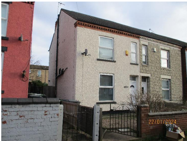
Front (south west) & side (north west) elevations.
